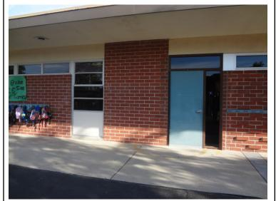
Photo - 1 Administration Building: Building 1 Administration building is made of brick masonry construction with a planar roof condition.
