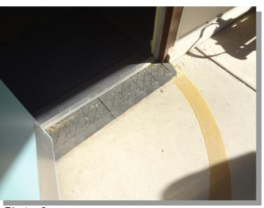
Photo -3 The building does not have current accessibility compliant thresholds
